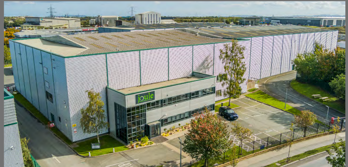
High Bay Logistics Portfolio, Northwest Business Park, Dublin
